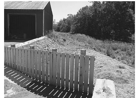
Silage Bunker -vegetated filter
